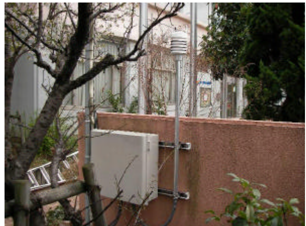
Figure 9. Installation of weather station at elementary school
