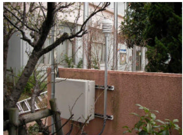
Figure 9. Installation of weather station at elementary school
