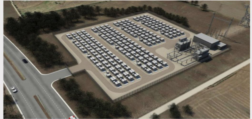
Above: Tesla's utility storage.
