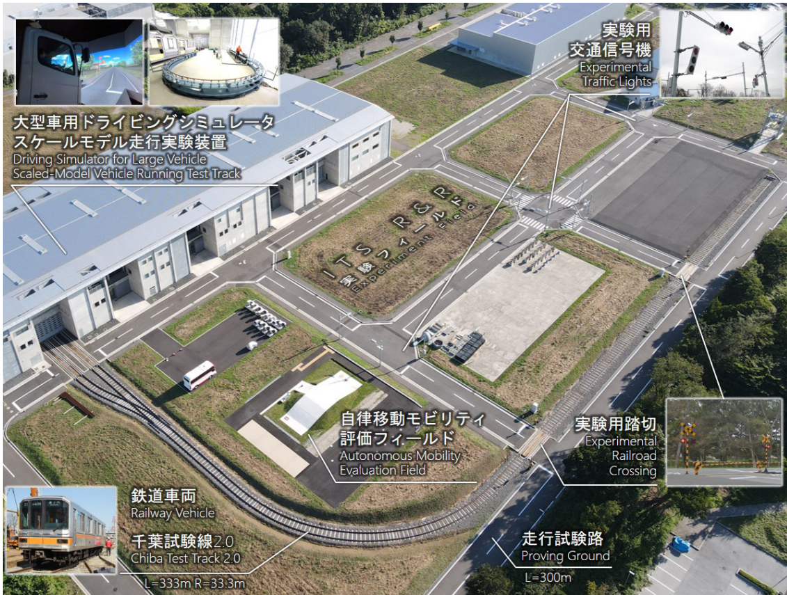
Fig. 6.9: Overview of the Kashiwa ITS R&R Test Field
