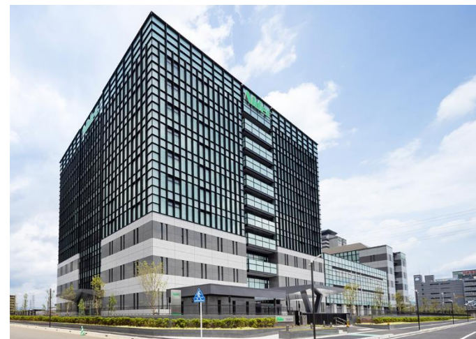
Nidec Central Technical Laboratory (Building C, Nidec Park, Muko-shi, Kyoto)
